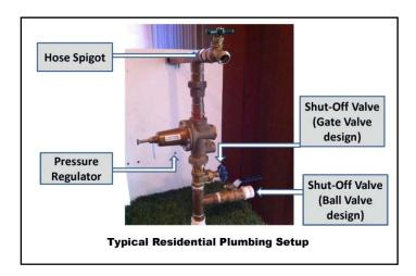
This should be the valve customers use first when turning off water to their house in the event of an emergency or plumbing repair. This valve can come in two designs: Gate Valve or Ball Valve. A word of caution, if this valve is not exercised (closed and opened slowly) at least once a year, it may not work correctly at a time of great need. If there is a problem with this valve, it is important to have a certified plumber make the repairs.
